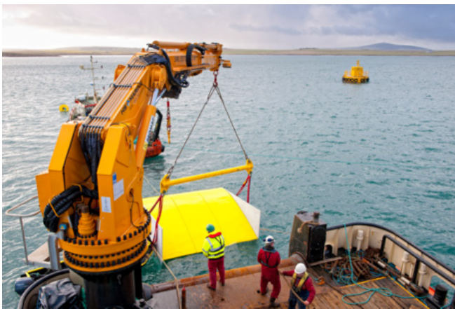
The example of tidal power plant installation
